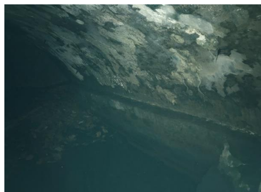
'Queen Anne's Well' showing brickwork arch detail. Note slate/tile inserts. The walls are very thick and of substantial construction
