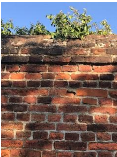
Wall showing English Bond and gabled capping
