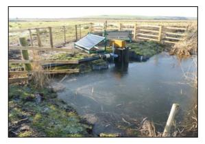
Three fish-friendly water pumps, each powered by three solar panels (nine panels in total) were installed on Wennington Marsh (part of RSPB Rainham Marshes nature reserve in Essex). These installations, together with associated ground works, happened during the winter of 2017 as an early success for Land of the Fanns. The pumps have since worked very effectively and helped the breeding productivity of key waders on the site, by maintaining invertebrate-rich wet areas, particularly
